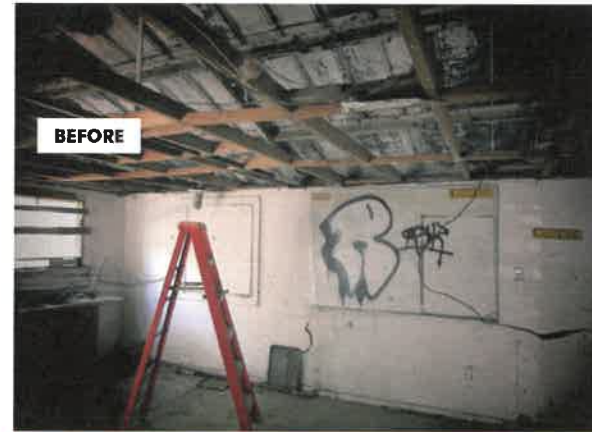
Waterworks Site Kitchen Restoration Project
