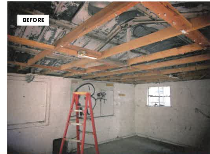
Waterworks Site Kitchen Restoration Project
